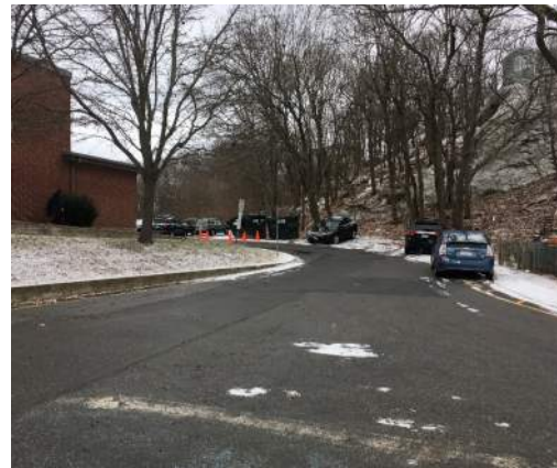
Accessible Parking not Located Near Ramp
