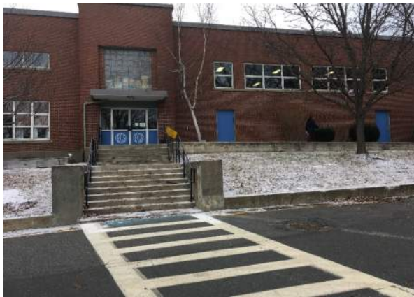
Incorrect curb cuts
