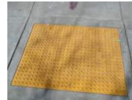
Accessible curb cuts with textured material
